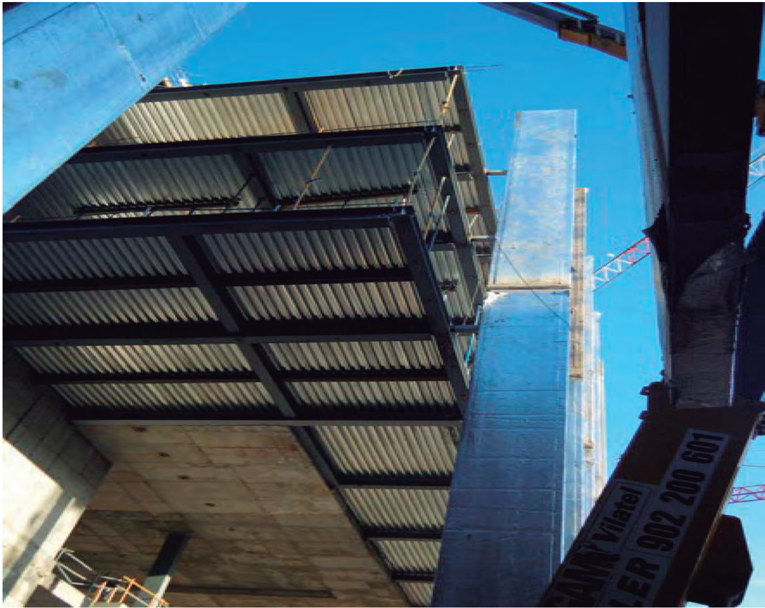
Connection of the structural box with the rib
