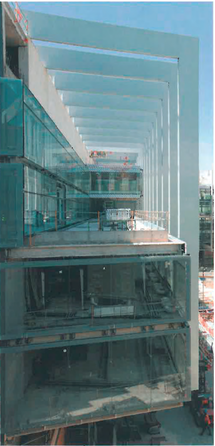
Connection of the structural box with the rib
