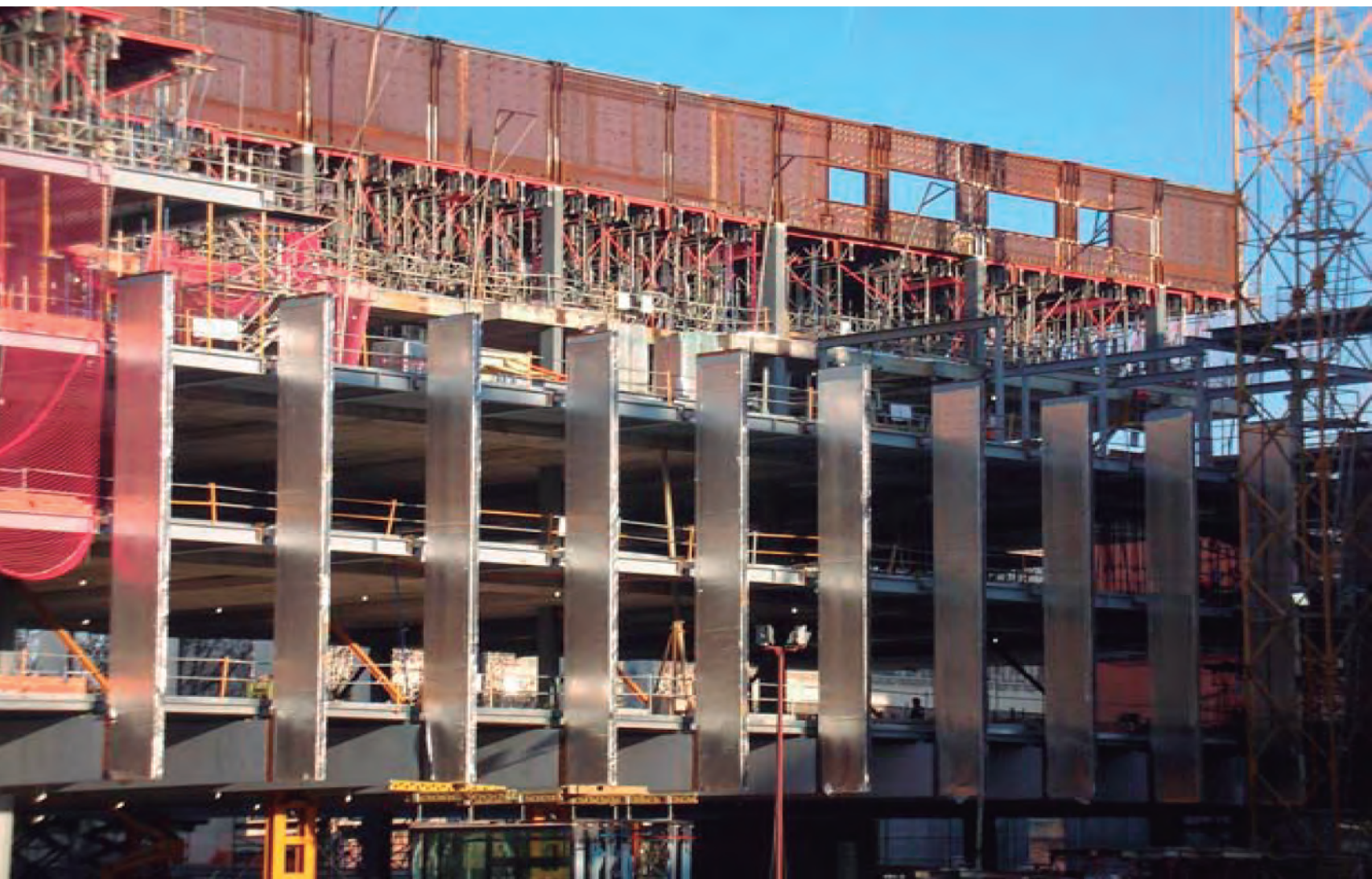
Connection of the post tensioned slab with the substructural frame
